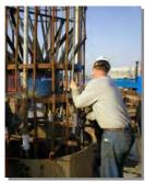
Installation of reinforcing cage with O-cell
